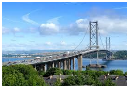
Firth Road Bridge
